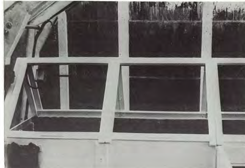
A propagation case showing rod thermostat and frame-warming cables.
